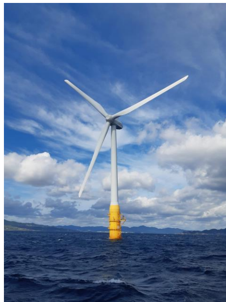
Figure 4: TODA Corporation ballasted spar near Goto Island, Japan.
